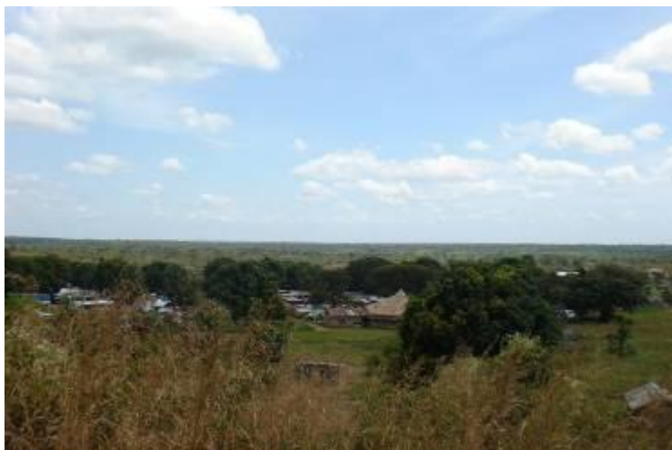
The small cross roads town of Lainya with cathedral central
